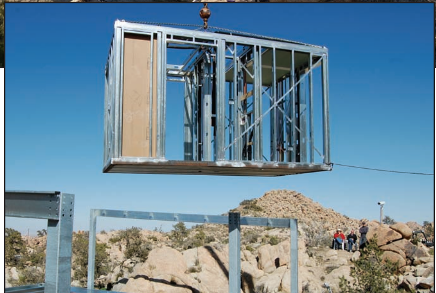
THE ALL-STEEL STRUCTURE WAS ASSEMBLED IN MODULES ON THE JOBSITE.
