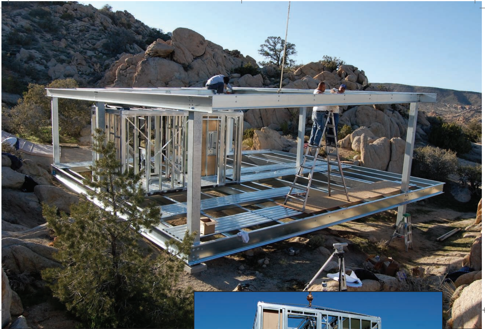
THE ALL-STEEL STRUCTURE WAS ASSEMBLED IN MODULES ON THE JOBSITE.
