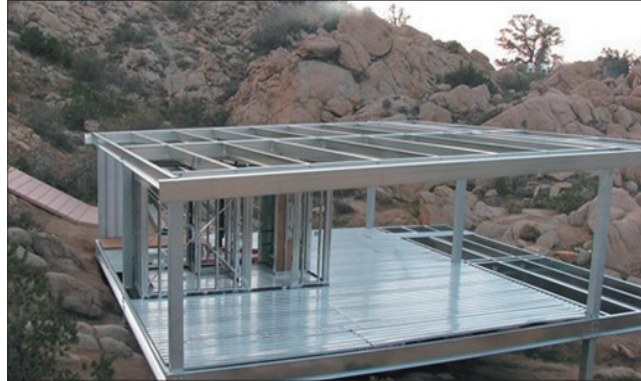
From start to dried-in in five days. Finished floor is polished concrete. The inner steel framed box shown is a craned-in “core module” with factory assembled electrical panel, principal plumbing, bathroom, water heater and HVAC system.
