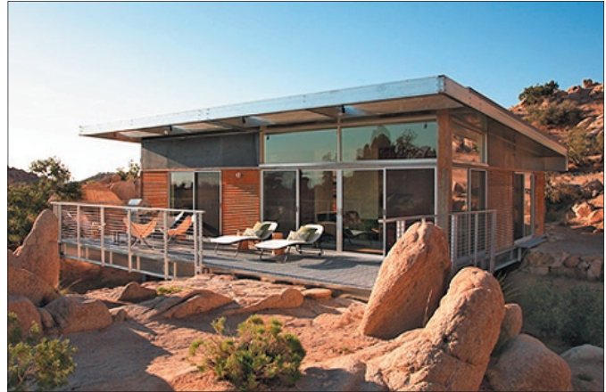
Blue Sky's Yucca House prototype: a kit house framed with cold-formed light-gauge steel. Up in six weeks, $246,000, ramping up for distribution and generating a lot of press.
